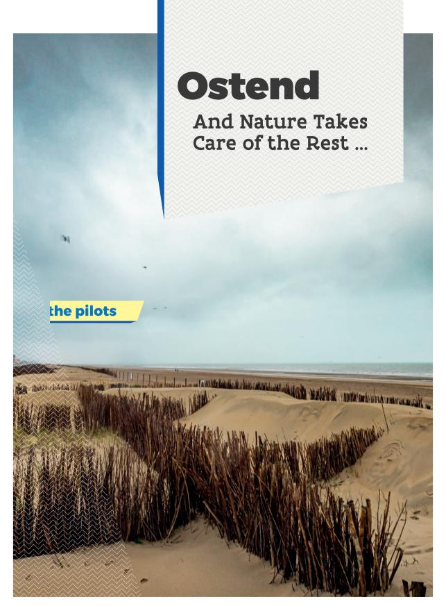
A dune-before-dyke ensures that the wind no longer blows the sand onto the tram tracks. The natural solution also offers other advantages: it creates valuable nature and the dune provides additional protection against sea level rise.
