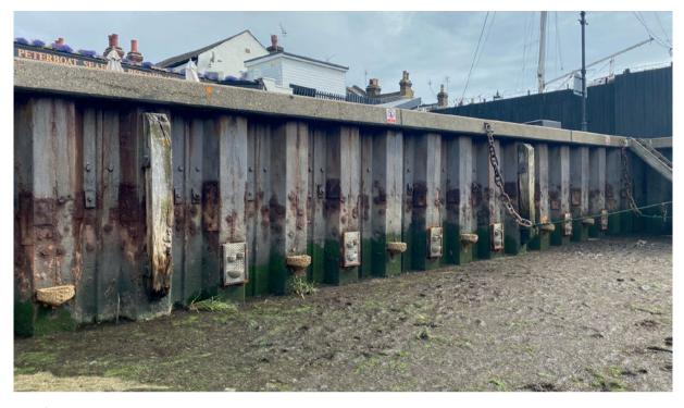
Vertipools and steel piling habitats. Small pools of low-carbon materials such as quarry waste provide an ideal substrate for marine life.
