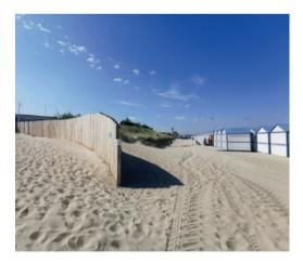
To create a natural sea defence high enough to protect Gravelines against sea level rise, a simple system of wooden fences was developed that hold back the sand being blown in.
